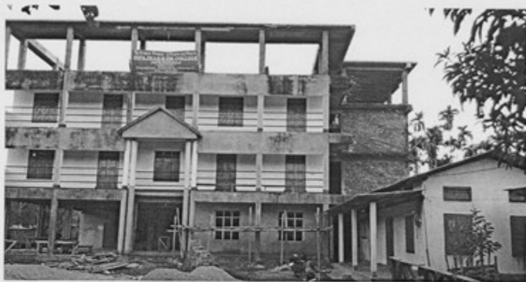
Front View of Building
