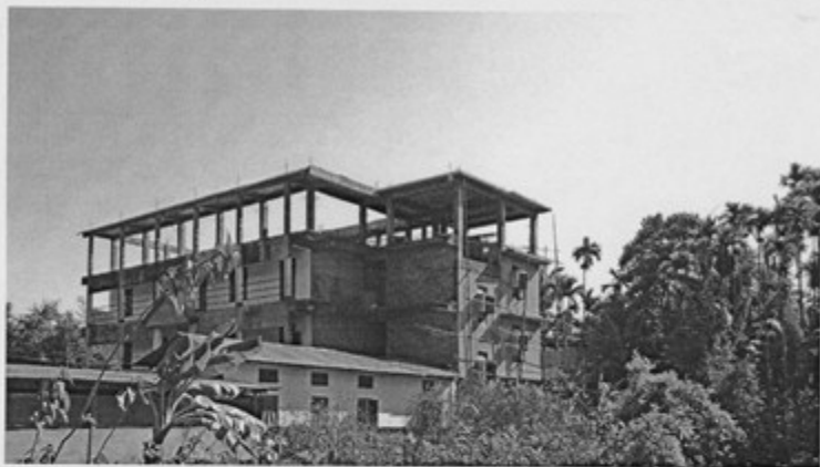
Rear View of the Building
